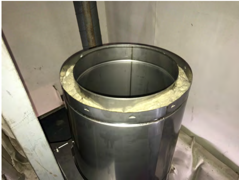
Female end of pipe segment with notches
